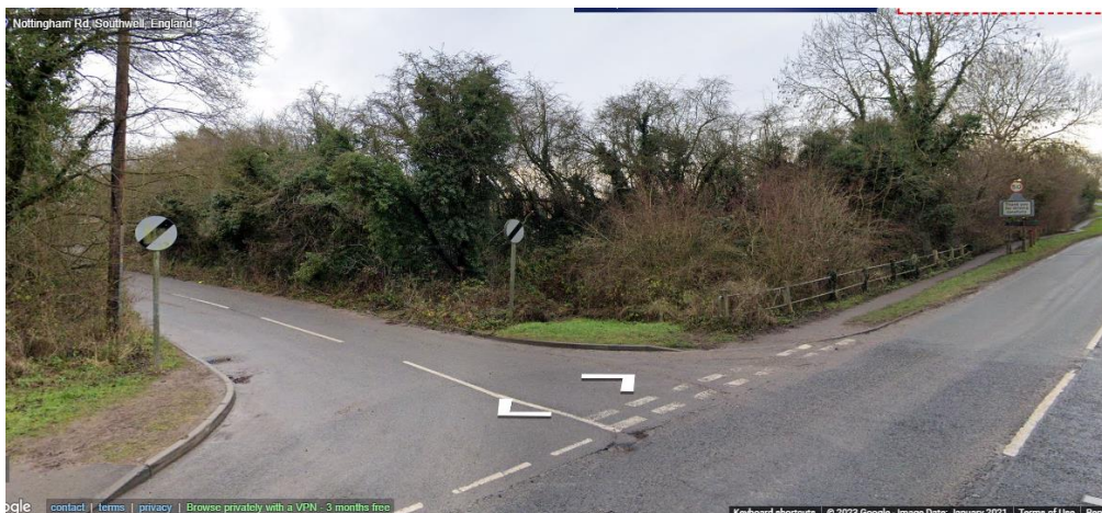
Figure 14: Current junction of Nottingham Road/Park Lane (courtesy of street view)
